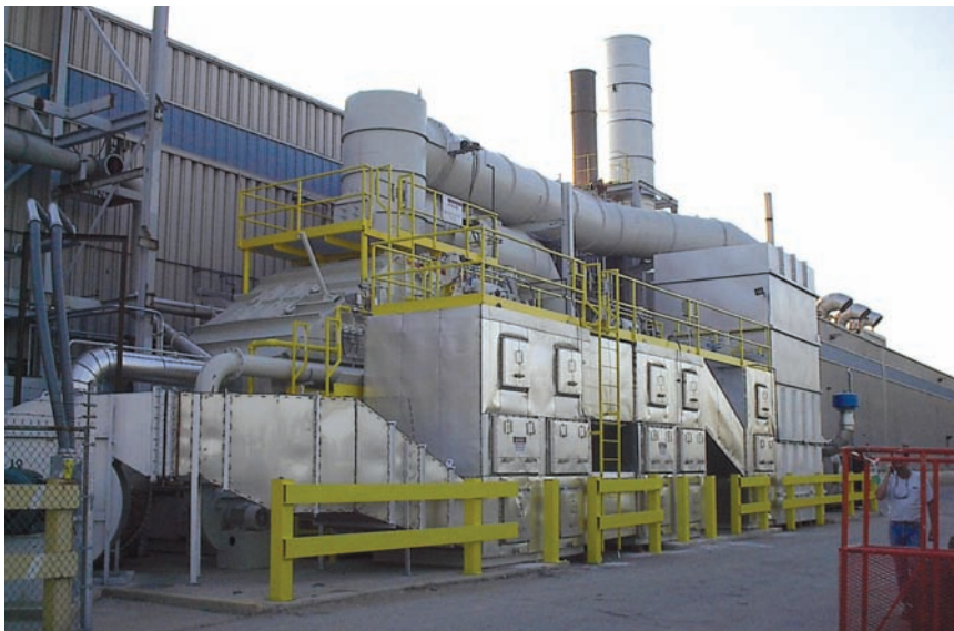
New oxidizer designs can deliver 95 or 96 percent heat recovery and a hot-gas bypass damper to deal with high VOC-loading periods.
