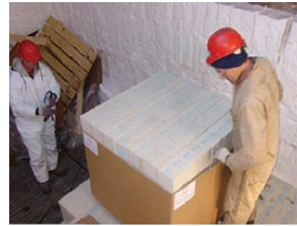
To improve primary heat recovery in regenerative thermal and regenerative catalytic oxidizers, consider increasing or changing the type of ceramic heat-recovery media.
